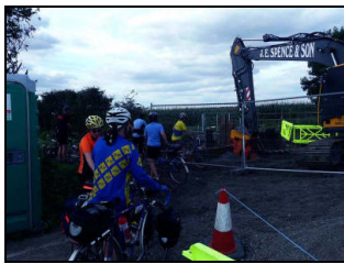
Road works near Scotter
