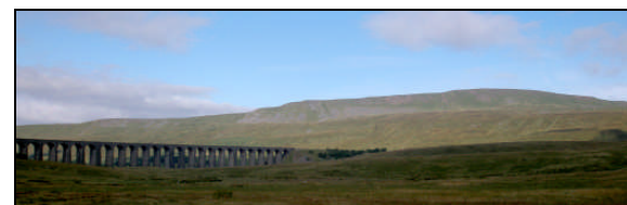
Ribblehead Viaduct and Wherside
